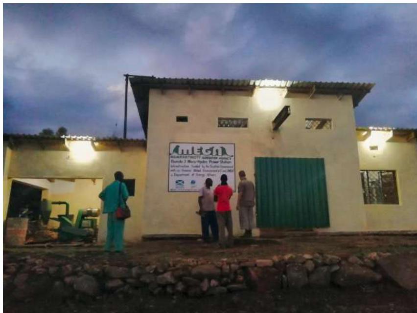
Power station at MEGA Bondo hydro plant
